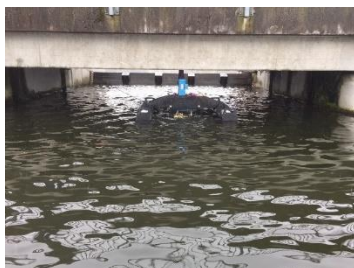
OLOID Type 400 with flow direction to the dam shutter
